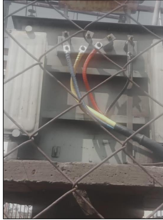
33KV Grid After work 300 mm. cable termination
