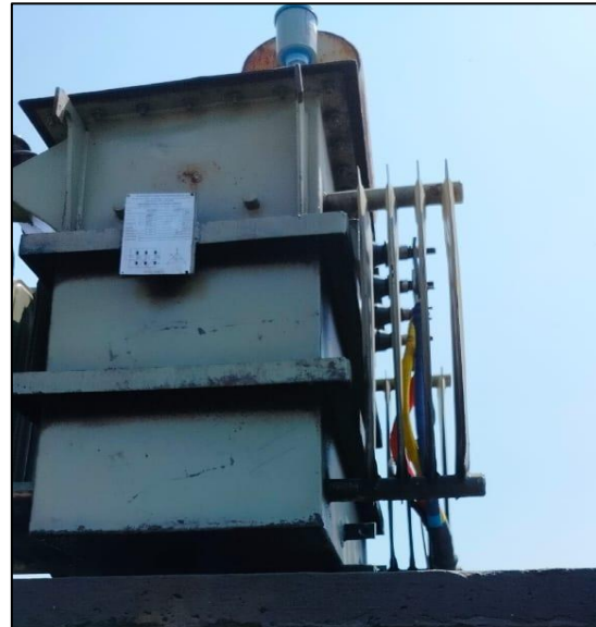
33KV Grid After work oil level and new Breather installed
