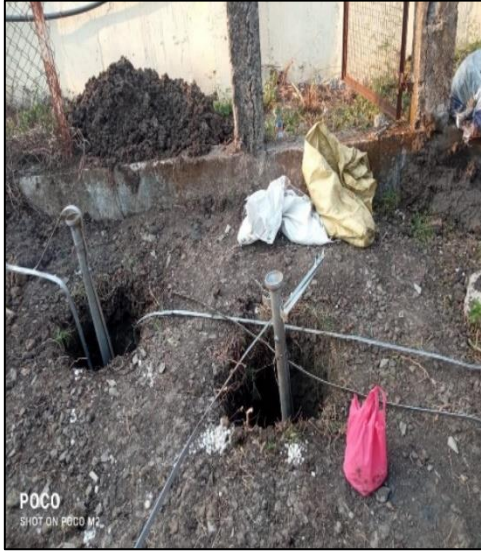
33KV Grid After work 07 Electrical GI earthing
