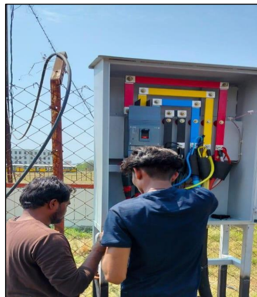
33KV Grid After work 300 mm. cable termination
