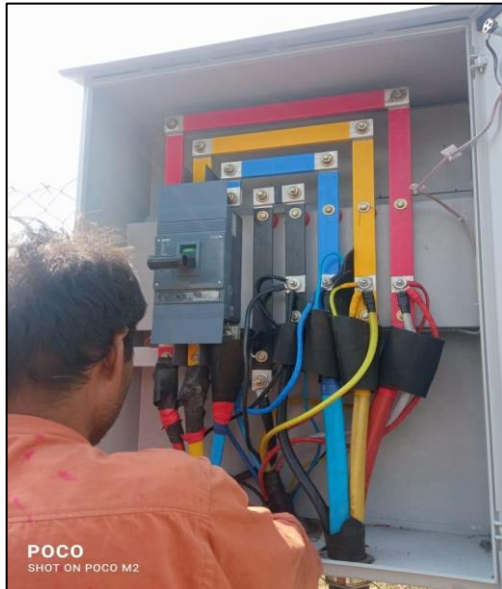
33KV Grid After work 300 mm. cable termination
