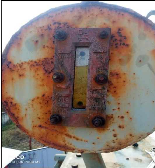
33KV Grid After work oil level and new Breather installed
