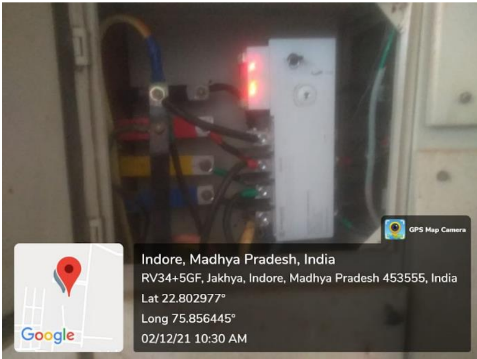
Figure.8: System for Automation of DG Set
