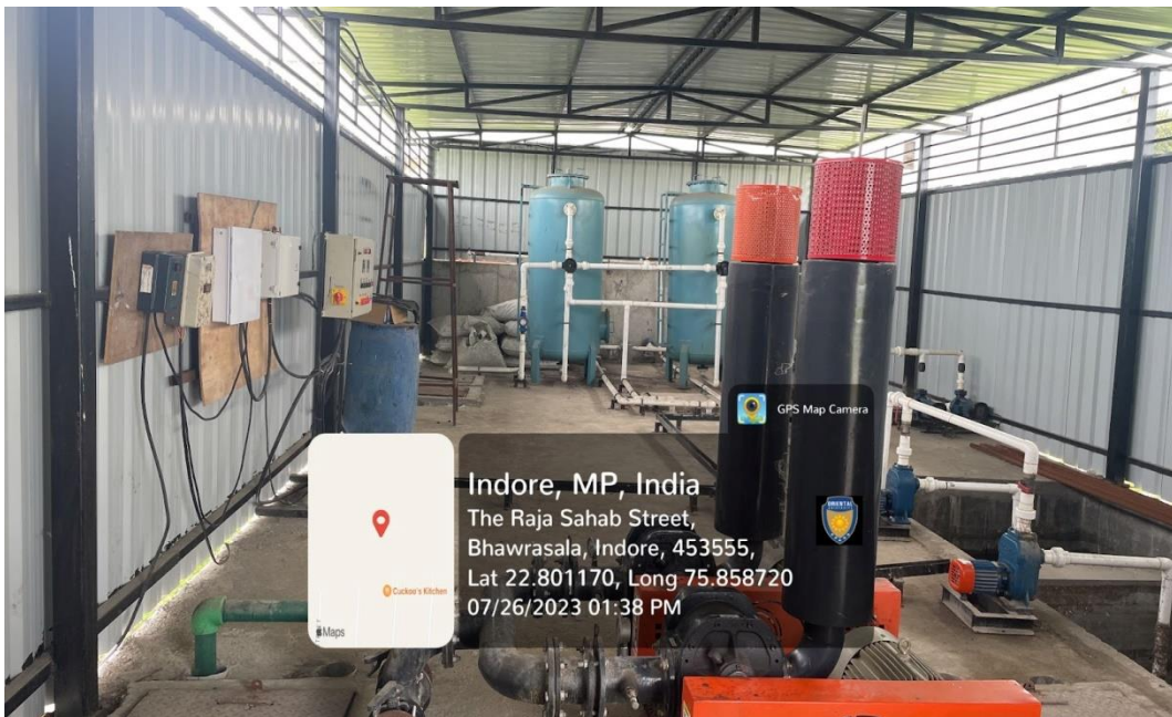
Figure.7: Geotag Photographs of Sewage Treatment Plant (STP)
